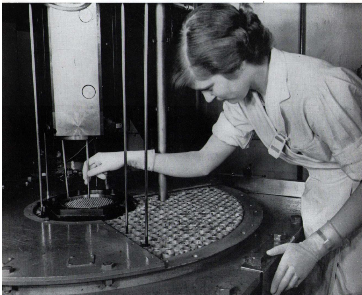
Loading a fuel element into Zephyr. This zero-energy fast reactor is fuelled with plutonium rods canned in nickel; the core is surrounded by a blanket of uranium in which more plutonium is bred. With Zephyr the first British experience of fast reactor operation was gained.
