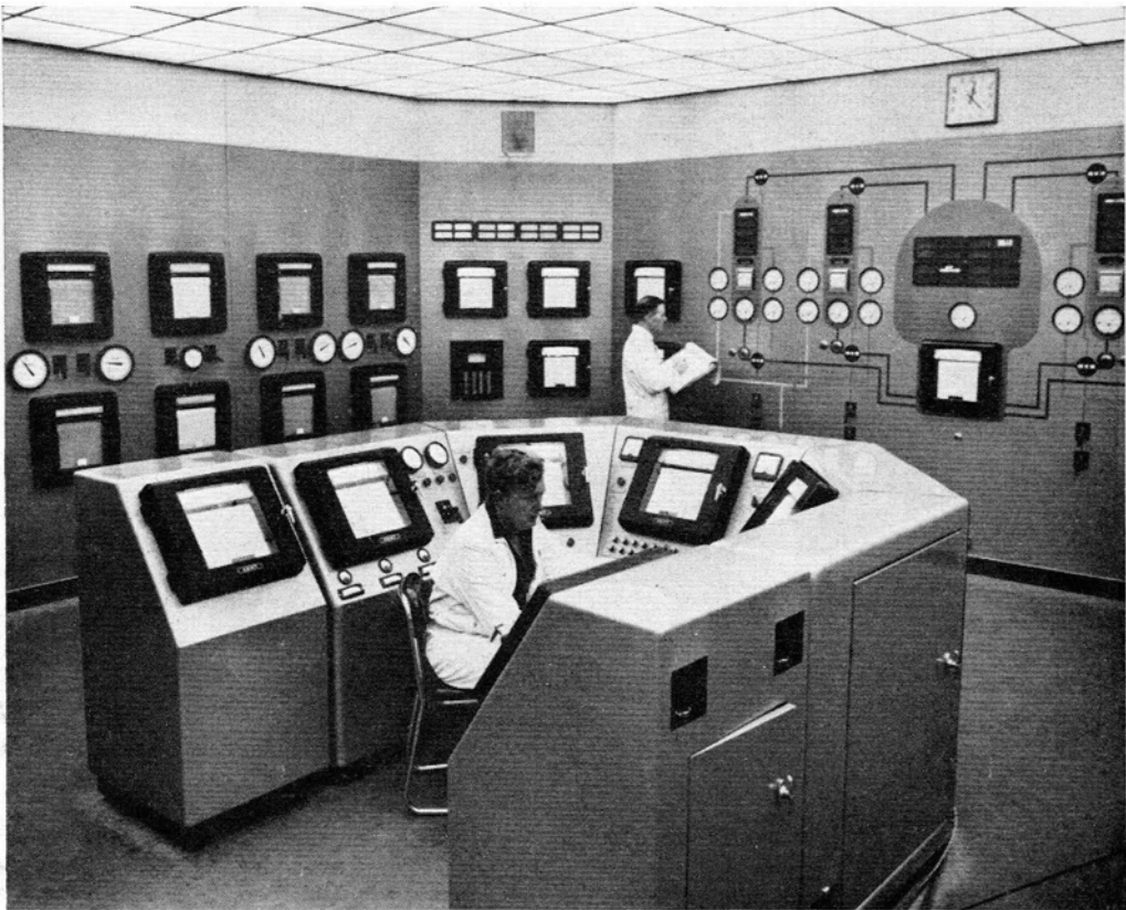
THE CONTROL ROOM of a Calder Hall reactor
