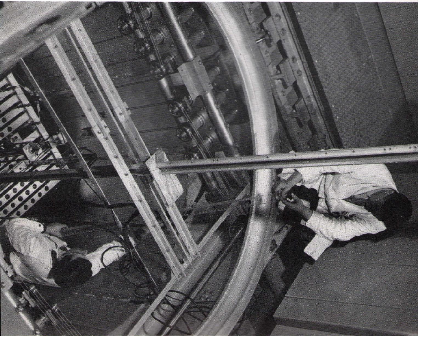
NEPTUNE zero-energy reactor: the inside of the reactor after the top shielding has been removed and the water moderator drained off
