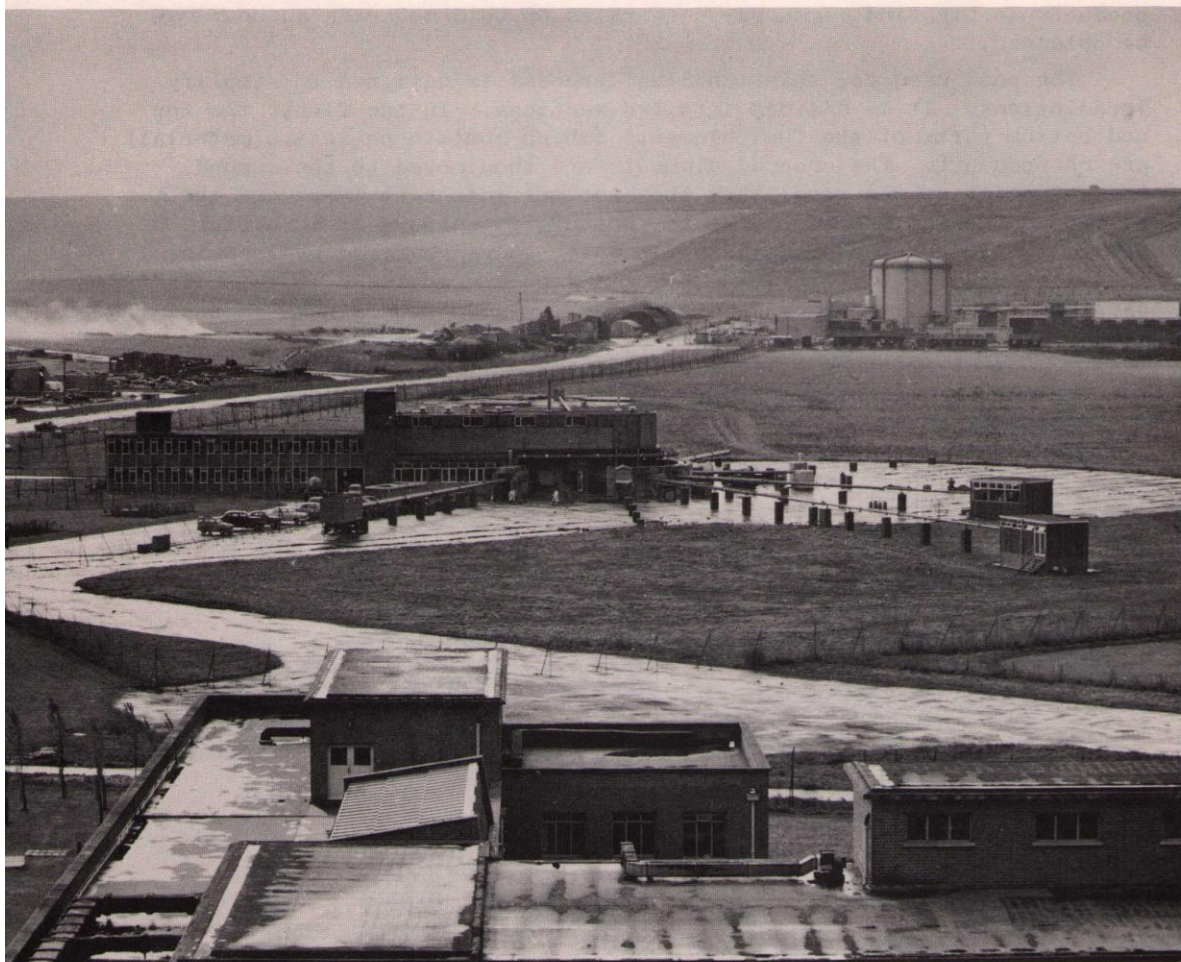
The neutron project building with flight tubes radiating from the target room
