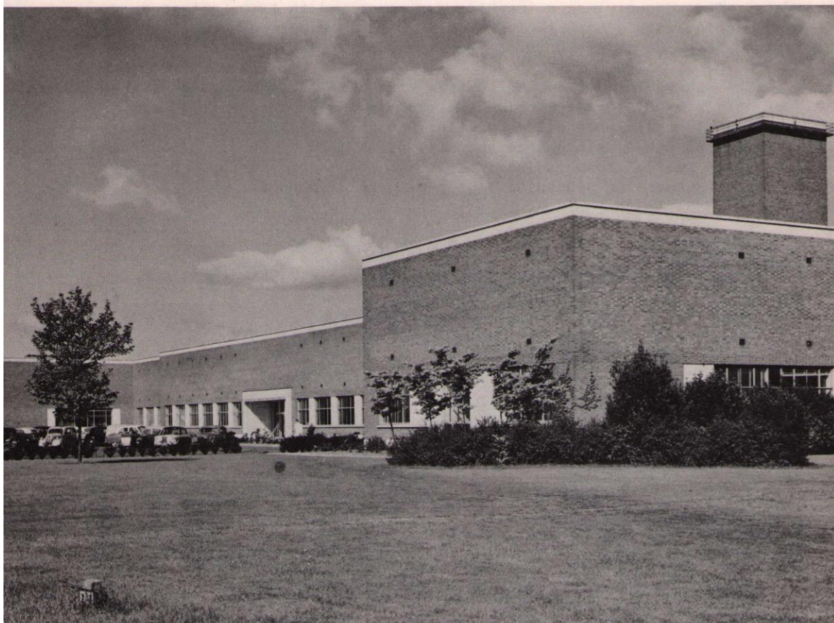
The radiochemistry laboratory, Building 220
