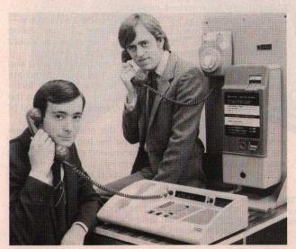
standard handset and control unit and operates independently of the British Telecom network. The main control unit is operated by teaching staff and connected to a call box in another room. To the pupil the system appears to be a normal telephone installation, but it can be closely supervised.
