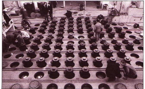
Pile cap of Number 1 reactor with control rod mechanisms and flux scanners in position.
