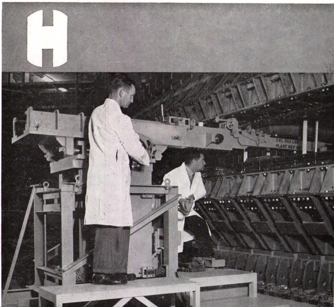
Installation of Upper Pole Piece for 'NIMROD' magnet at Rutherford Laboratory
