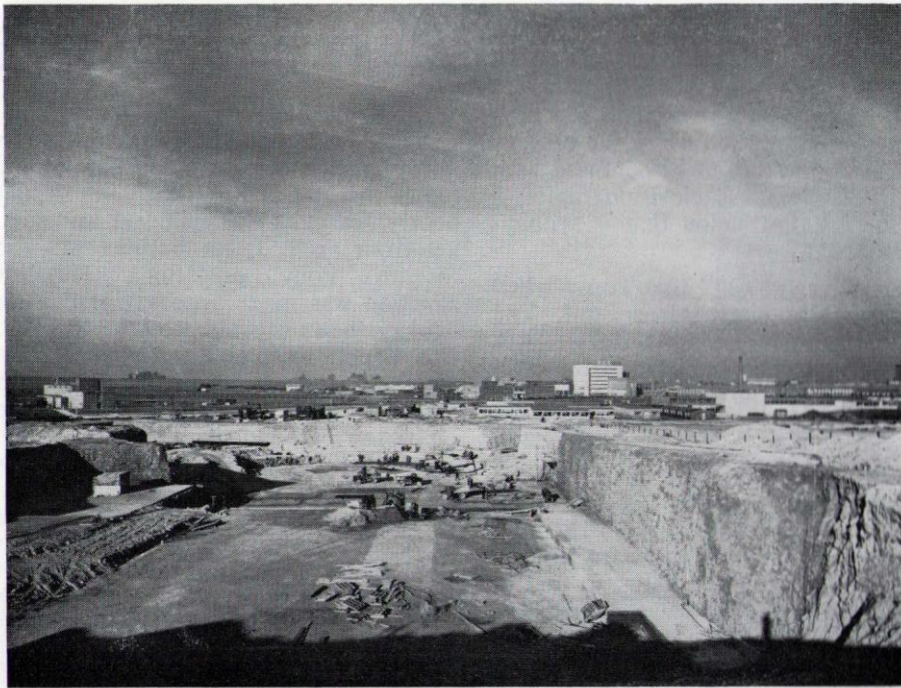
Early days: Excavation work for Nimrod.
