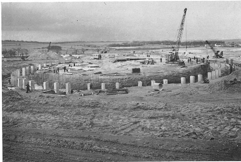
Nina magnet foundations
