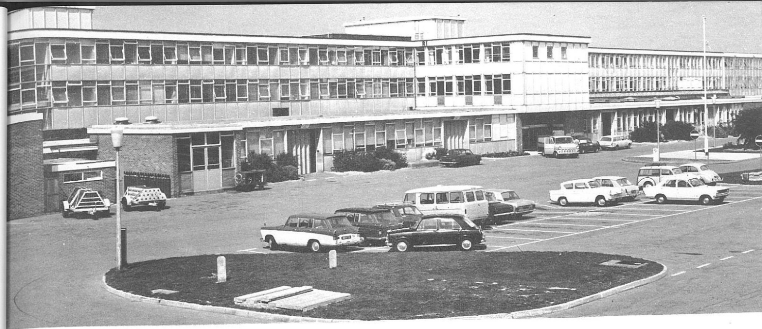
Figure 136. Building R1. Main office and laboratory block.
