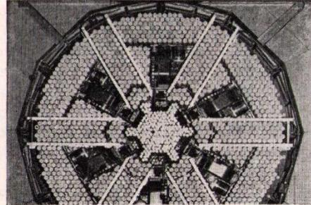
**7. ZEUS** (Harwell). Zero Energy Uranium System. This 100-watt research reactor began working in 1955. It is an uncooled fast reactor with a large highly enriched uranium core (the same size as the Dounreay reactor core) and a natural uranium blanket for breeding studies.
