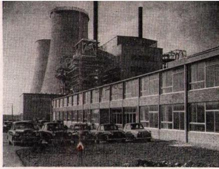
**2. CALDER HALL** (Cumberland) power reactor is to operate in October, 1956. In the complete station there are two graphite moderated reactors, cooled by carbon dioxide under pressure, and contained in mild steel pressure vessels 40 ft. in diameter and 60 ft. high housed in thick concrete biological shields. Outside these stand the huge cylindrical heat-exchangers, four to each reactor.
