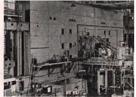
**4. BEPO** (Harwell). British Experimental Pile in continuous use since 1948. Another graphite moderated air-cooled reactor used primarily experimentally but also for making isotopes. Its power is limited to 6,500 kilowatts (dissipated as heat in the cooling air), its core consists of 850 tons of graphite and the full uranium metal load is 40 tons.
