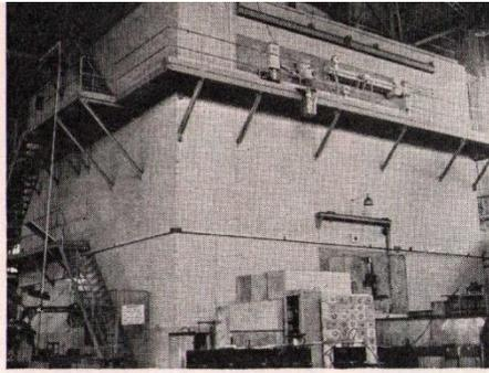
**3. GLEEP** (Harwell) Graphite Low Energy Experimental Pile. This graphite moderated air-cooled reactor has been in continuous use since 1947 for general experimental purposes. Its maximum operating power is limited to 100 kilowatts (it normally runs at much less) and it contains 505 tons of graphite, 12 tons of uranium metal and 21 tons of uranium oxide.
