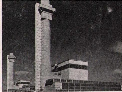
**1. WINDSCALE** (Cumberland) two thickly shielded plutonium production reactors operating since 1950. Each consists of an octagonal prism of graphite, pierced by a large number of horizontal channels in which are laid rows of uranium rods. Every rod is sealed in a finned, tightly fitting aluminium can and the heat produced in the nuclear reactor is removed by atmospheric pressure air.
