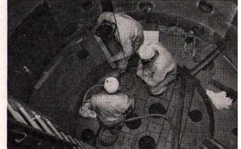
**8. DIDO** (Harwell). This 10,000 kilowatt high flux materials testing reactor should be worked up to full power by Christmas. Another heavy water moderated-aluminium tank reactor, it will have the highest neutron flux in Western Europe and be used for research and tests on fuel systems.
