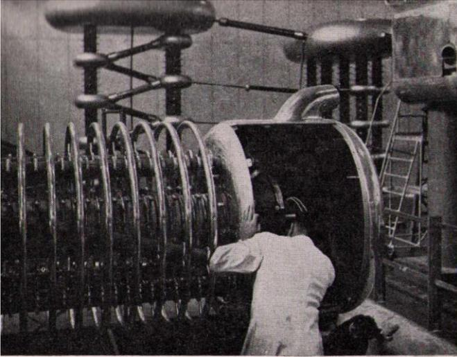
The 500,000 Electron volt proton injector at Harwell.
