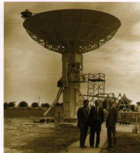
1979 The newly formed RAL director general Dr Godfrey Staffor, together with Dr Geoff Manning, director, Rutherford (left) and Dr John Houghton, director, Appleton (right) stand in front of the new IRAS dish, a 12m diameter, fully steerable S-Band antenna from NASA, constructed at RAL.
