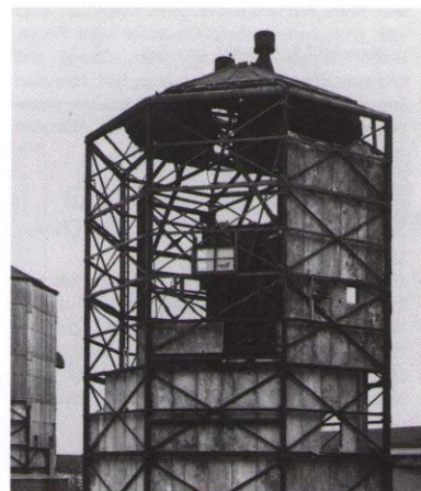
One of the three navigational training towers, known as 'The Harwell Box' used by the RAF for aircraft training to simulate engine failures, enemy aircraft attack and celestial navigation. The gunner had to follow the movement of a spot of light with another light which was fixed to the gun mounting in his turret. It was in a fall from the top of one of these towers that the first Harwell fatality occurred.
