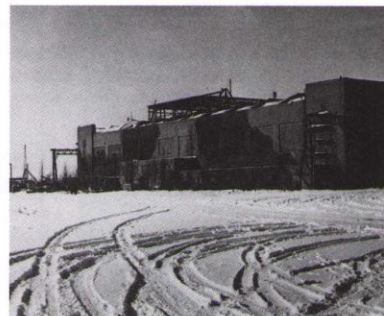
Hangar 10 in the snows of Winter 1947. The recently raised roof to accommodate the BEPO reactor can be seen.
