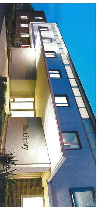
The 1950s architecture has been successfully combined with contemporary office design.
