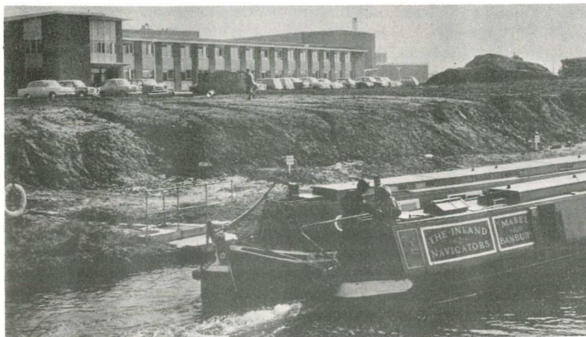
View across the canal of the laboratory and office block
