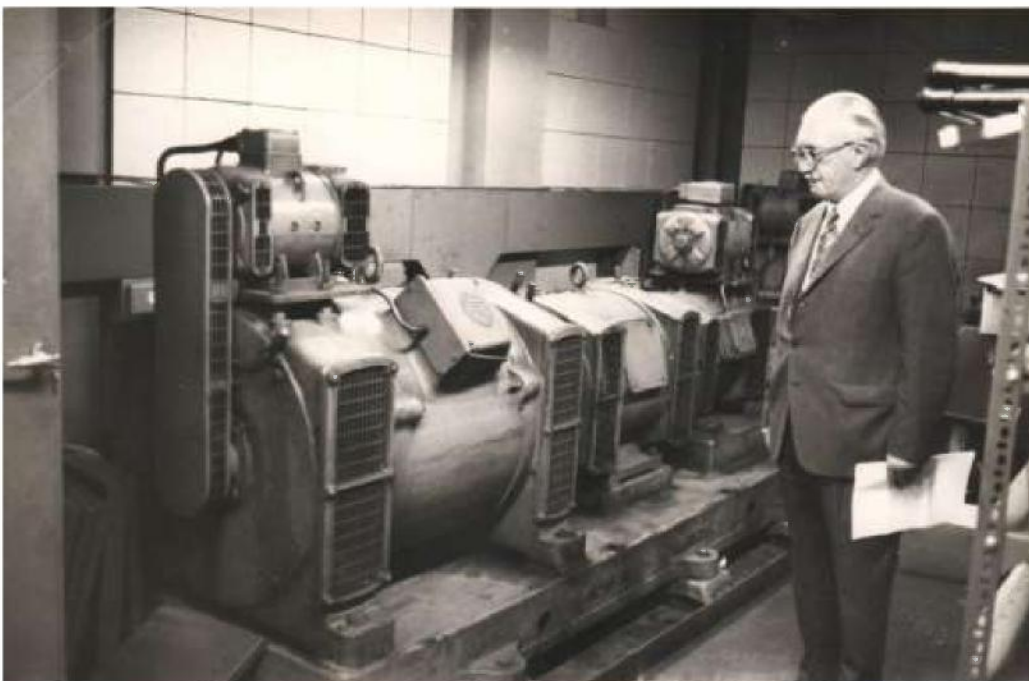
These motor alternators, of which there were three, supplied the power to the computer. One set was a stand-by. There was a separate small set supplying 80 cycle current to drive the four magnetic drums.
