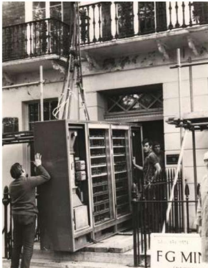
A view of one of the cabinets being taken through the front door. The building in which ATLAS was housed is scheduled as a building of historical interest and great care had to be taken not to damage the balcony or the fabric of the building
