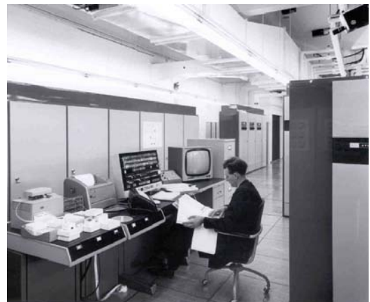
Storage and engineers’ console
