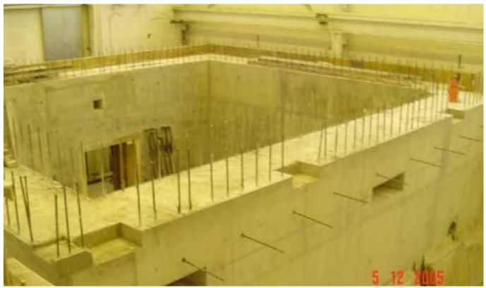
Target Area 3 bunker from the south east corner showing the metre-thick concrete walls, December 2005. The roof of TA3/floor of LA3 has yet to be added so you can see the entrance door to the bunker.
