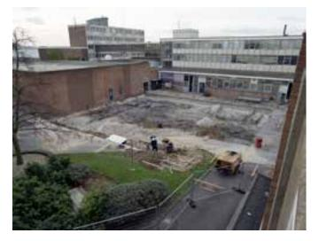
Ground work begins outside R1, digging up what used to be the Director's car park. The new building was approximately 21.5m x 24.5m in size, consisting of a brick faced external skin, 30 cm thick concrete radiation shielding walls, and an aluminium skin roof.
