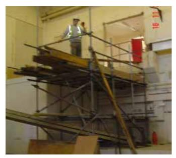
Build-up of shuttering for the TA3 bunker. The doorway hanging in mid-air is the door into Laser Area 3.
