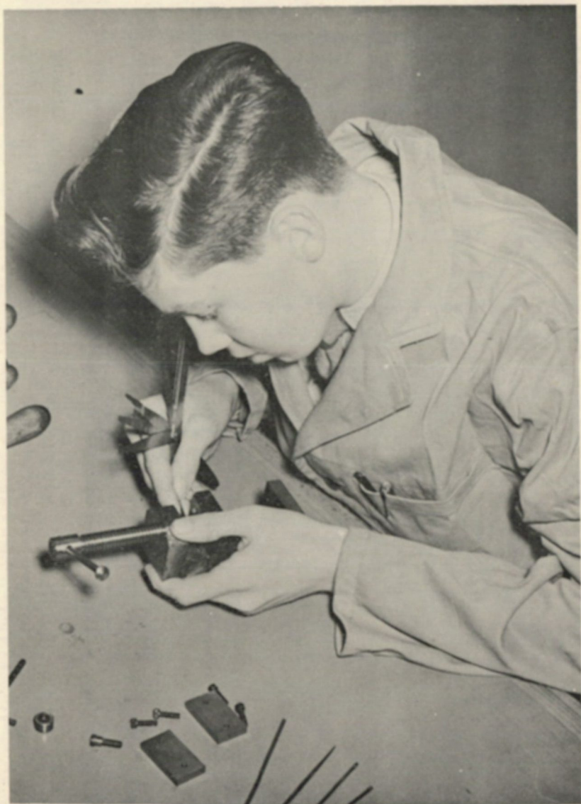
Having machined all the details himself, this first year apprentice is now checking the accuracy of his work as he fits the parts of his vice together.
